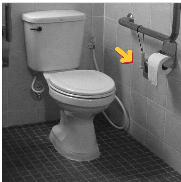
Fig. 35: Emergency system for restrooms / toilets
